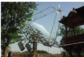
Example of renewable energy application for steam generation at Akshar Dham temple, New Delhi for community cooking
