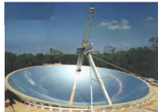
Example of renewable energy application for steam generation at Akshar Dham temple, New Delhi for community cooking
