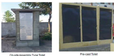
On-site Assembly Type Toilet
